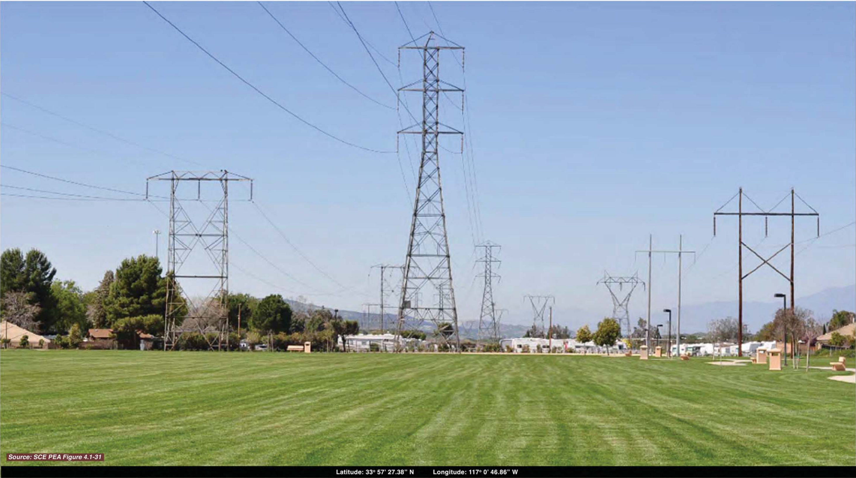
This image presents the Existing View to the northwest from KOP 6 at the east end of Stetson Community Park , in the City of Beaumont. This view encompasses a residential ROW park setting and a portion of Segment 4, just east of I-10. Three transmission lines pass through this residential development, creating a ROW that has been converted to a community park. KOP 6 Stetson Community Park Existing View SCE West of Devers Upgrade Project CEQA EIR / NEPA EIS Visual Resources Figure D.18-13A
