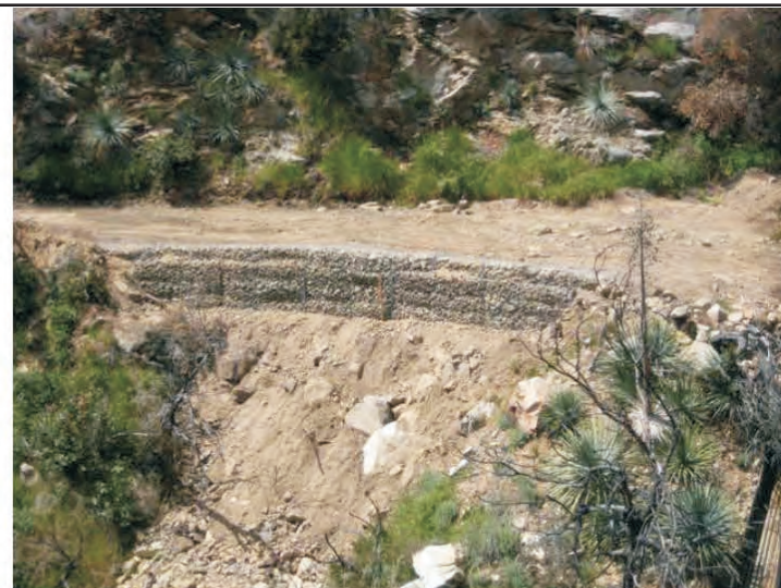
Typical gabion wall.
