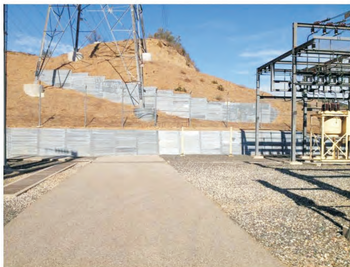
Typical soldier pile wall.
