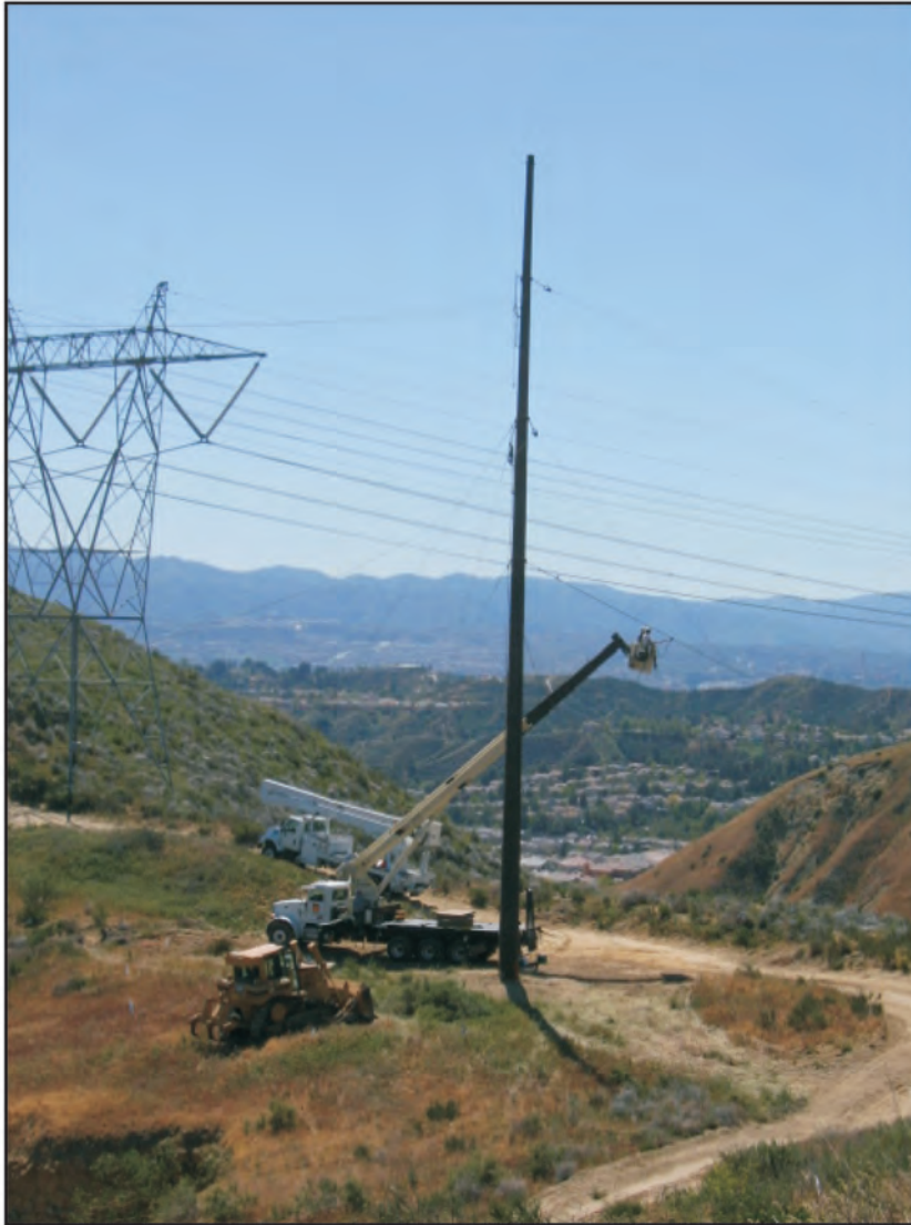
Photo 1. Wire installation on a shoo-fly pole.
