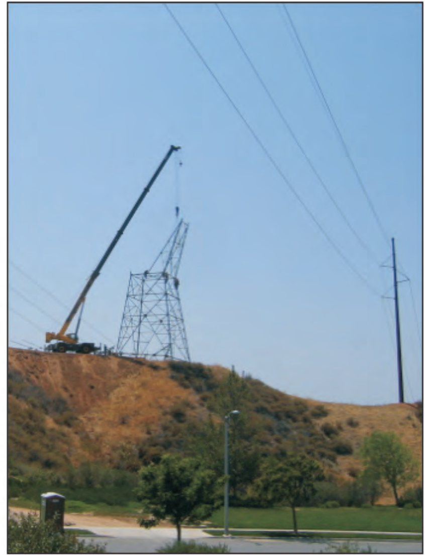
Photo 2. Shoo-fly in use during 220 kV tower removal.
