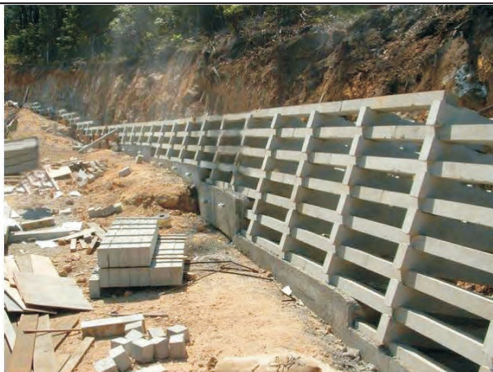
Typical concrete crib wall.
