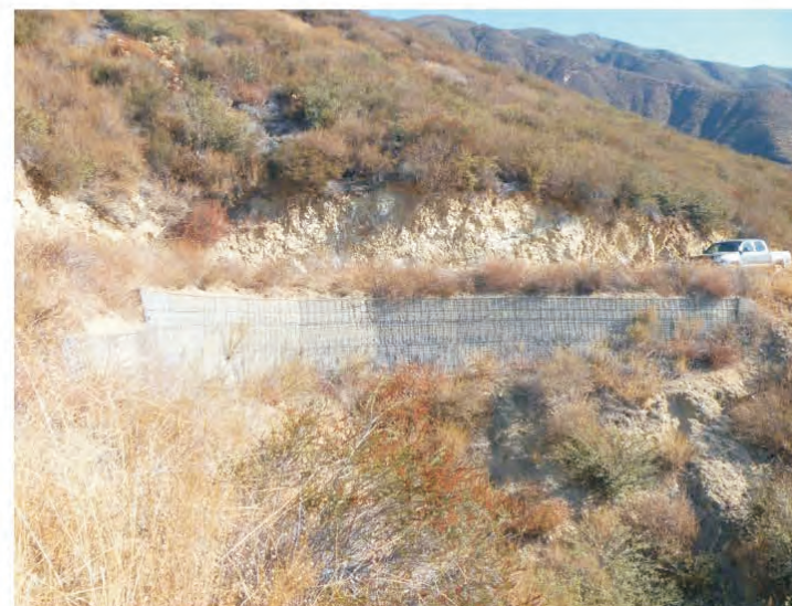
Typical welded wire wall.
