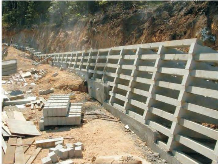
Typical concrete crib wall.
