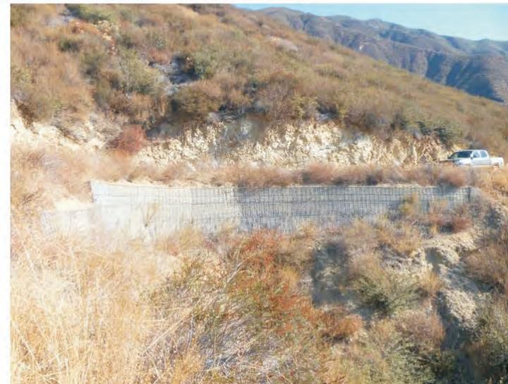
Typical welded wire wall.
