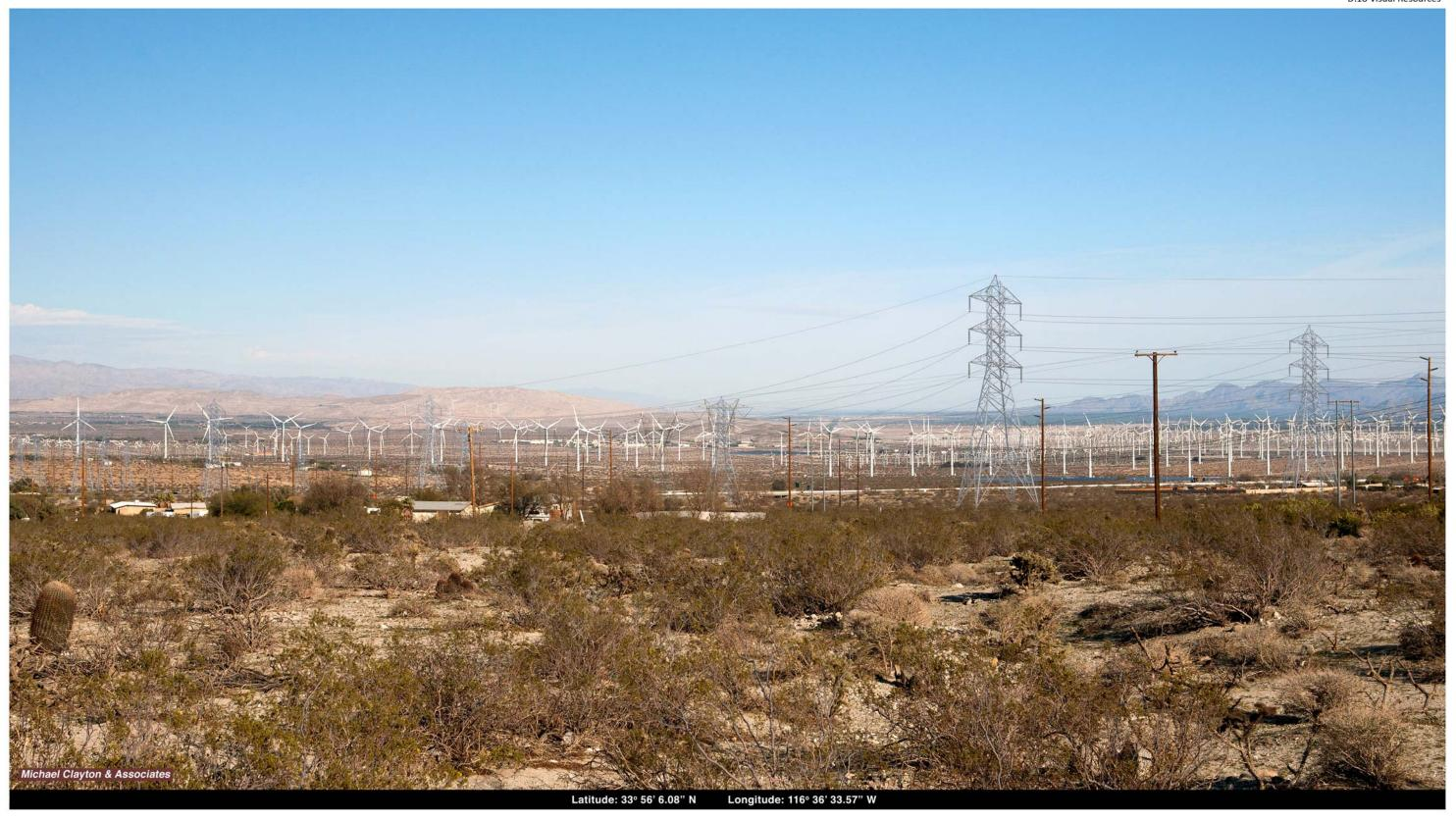
This image presents a **Visual Simulation** of the Proposed Project from **KOP 16**, on **Painted Hills Road**, immediately east of Verbena, west of SR 62. This simulation illustrates the replacement of three existing transmission lines of different design and size, with two transmission lines of greater height but identical design. As shown in the simulation, the new structures would be slightly more prominent due to greater heights.
