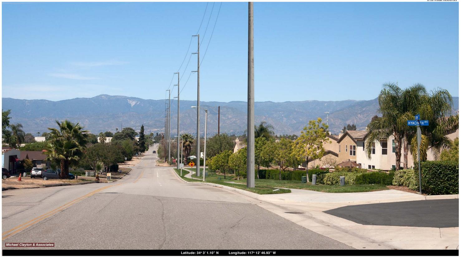
This image presents a **Visual Simulation** of a portion of the Proposed SB-Redlands-Tennessee overhead 66 kV subtransmission line, from **KOP 18** on **Iowa Street**, in the City of Redlands. The simulation illustrates the introduction of vertically prominent, light-weight steel poles into the suburban landscape along Iowa Street. As shown in the simulation, the new structures would be visually dominant features in views from Iowa Street and the adjacent Cottage Lane residential subdivision.
