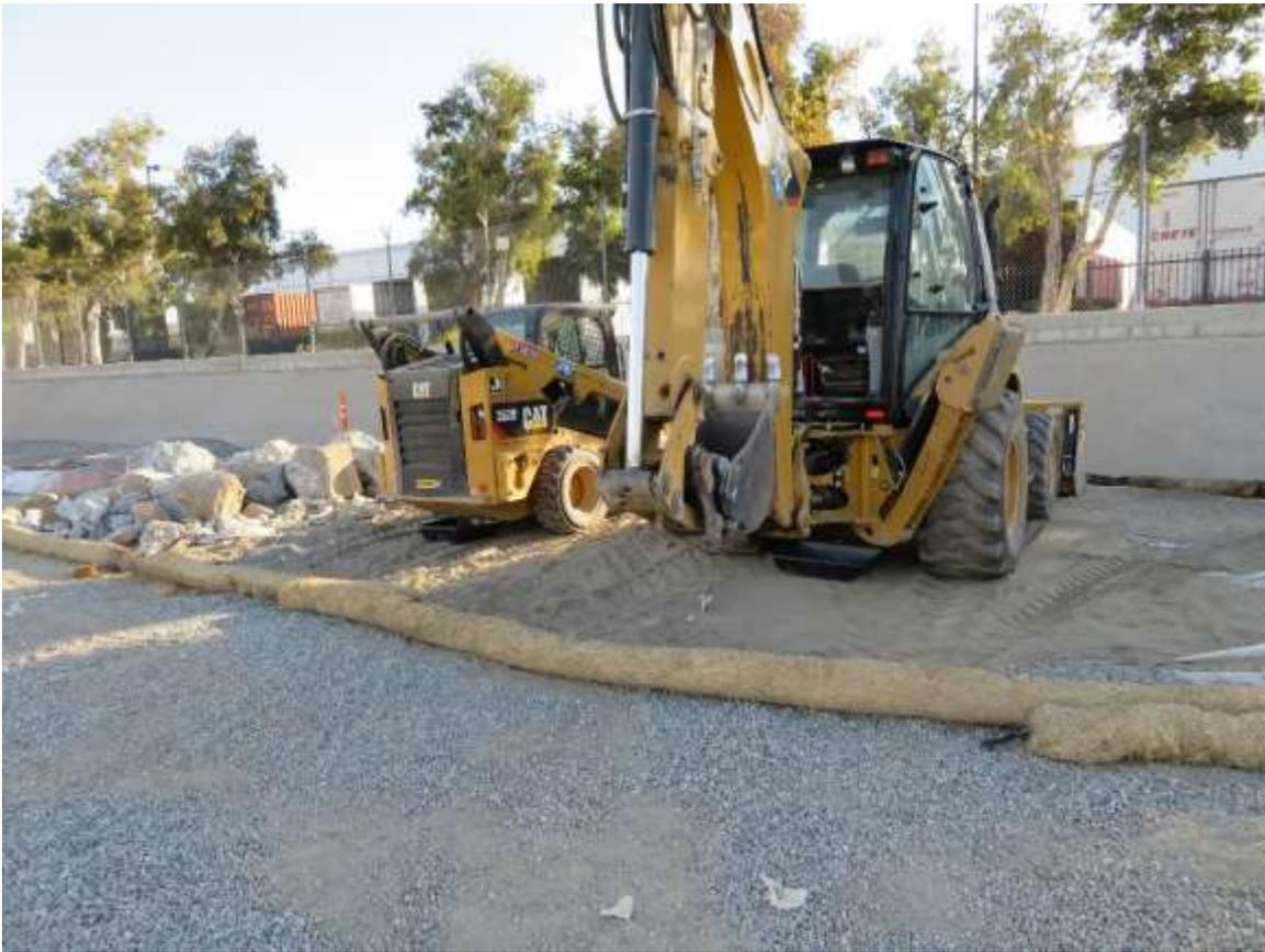
Figure 3 – Straw wattles were installed around the remaining soil stockpile in the material storage area, October 11, 2017.
