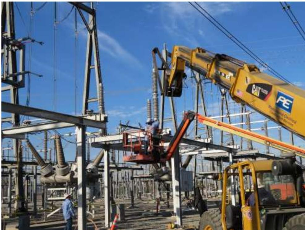
Figure 2 – New insulators were installed on the new switchracks, October 11, 2017.
