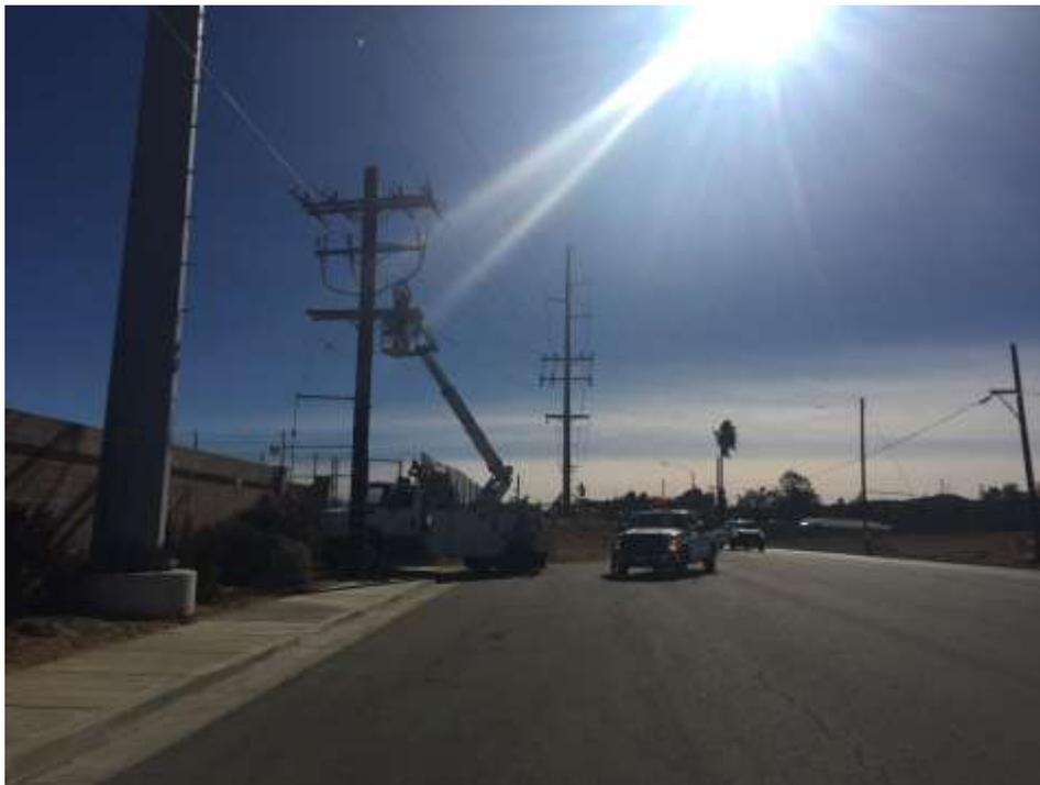
Figure 4 – SCE telecom crews installing fiber onto existing poles outside of the Maraschino Substation for the associated telecom alignment, December 8, 2017.
