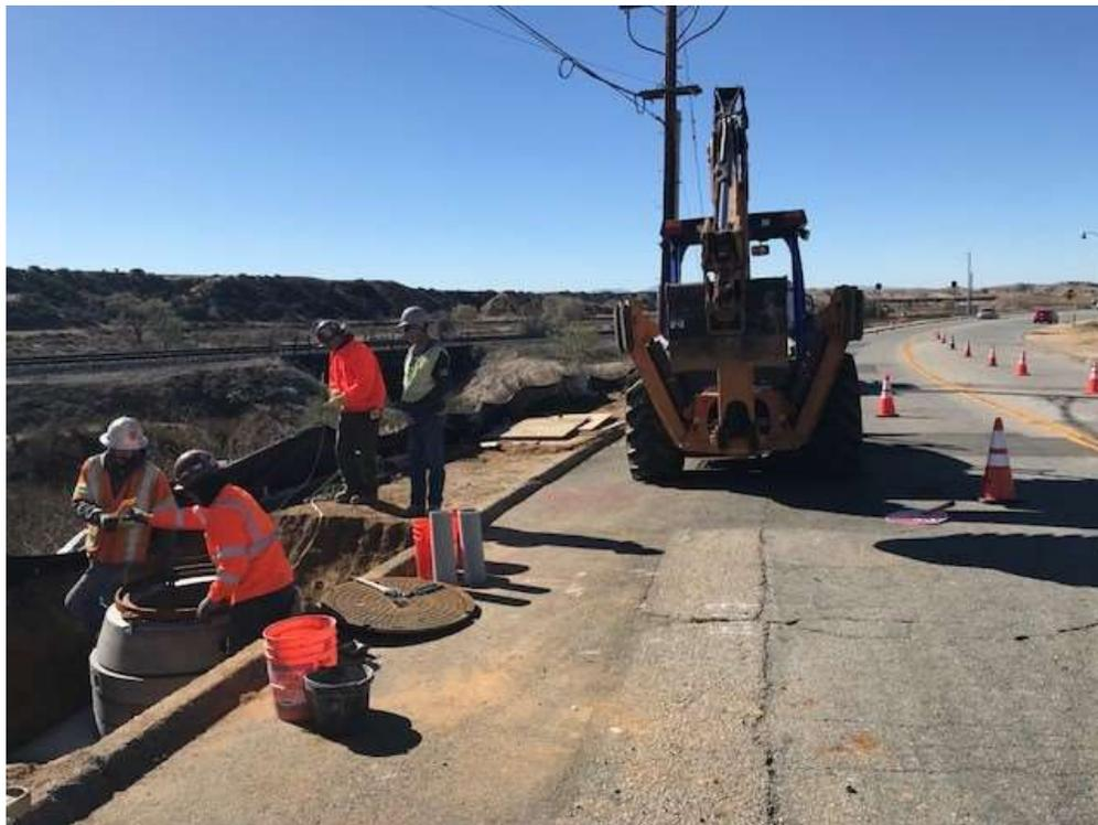
Figure 2 – W.A. Rasic crew excavating manhole during conduit installation along Oak Valley Parkway (January 22, 2018).
