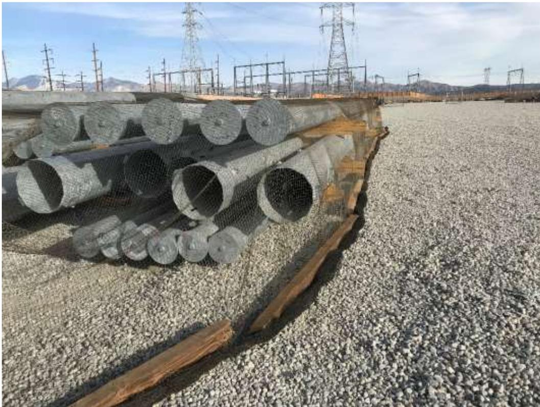
Figure 5 – Cribbing used to secure exclusionary bird netting at Devers MY (March 8, 2018).
