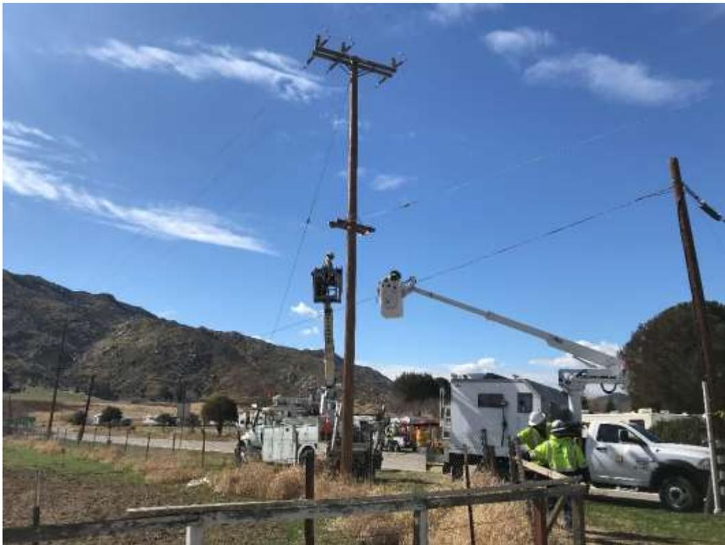
Figure 6 – SCE crew installing "flying corner" at intersection of Old Idyllwild Road and Wesley Street (February 21, 2018).
