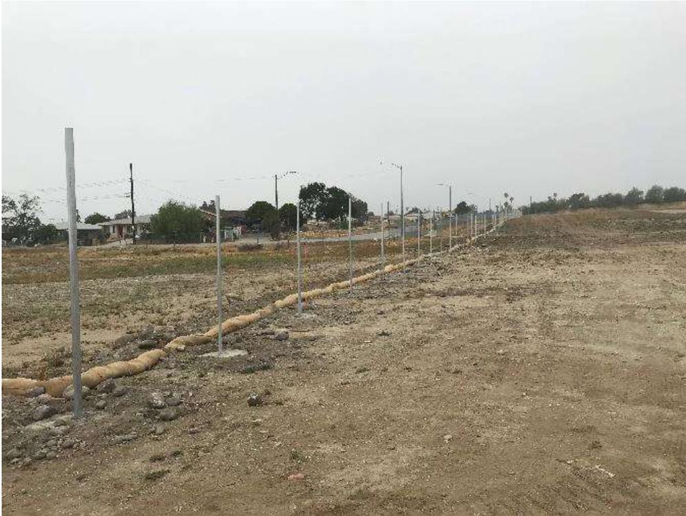
Photo 1 – Installing poles for perimeter chain link fencing at Match MY (May 24, 2018).
