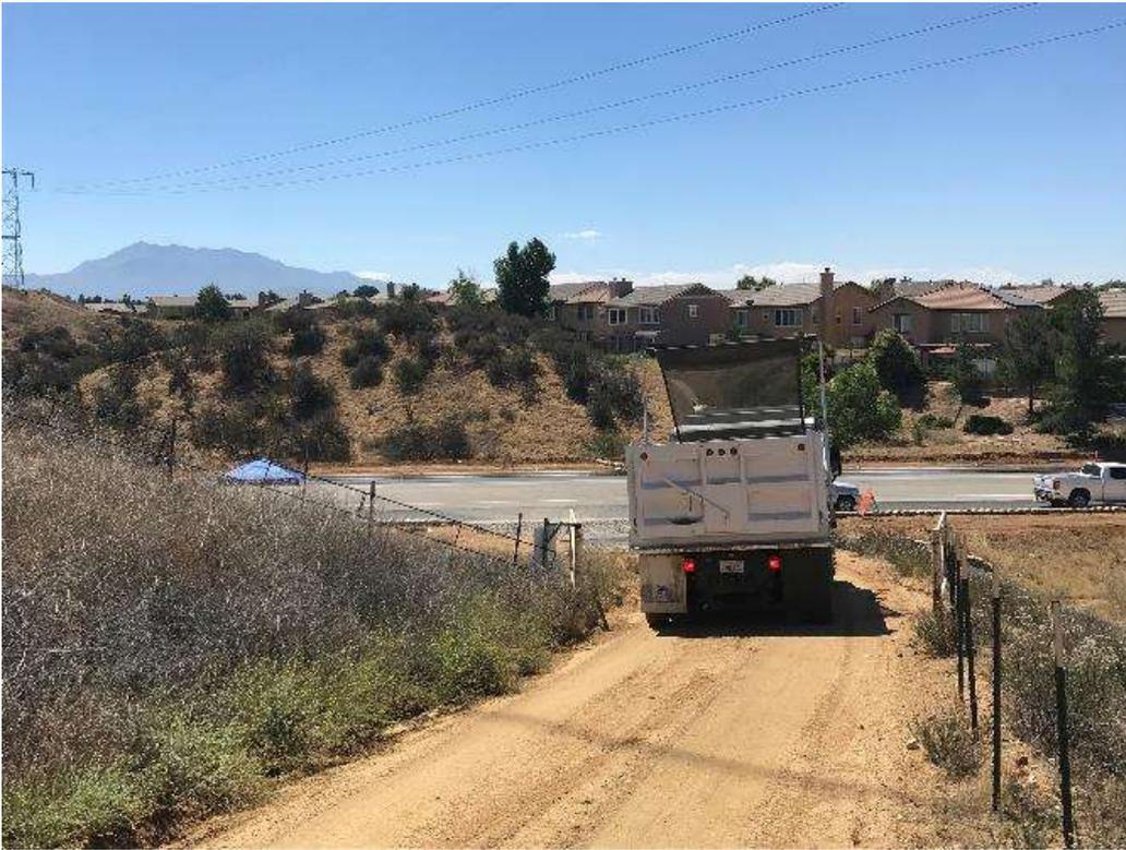
Photo 7 – Haul truck properly covering load prior to leaving Segment 4 (June 14, 2018).
