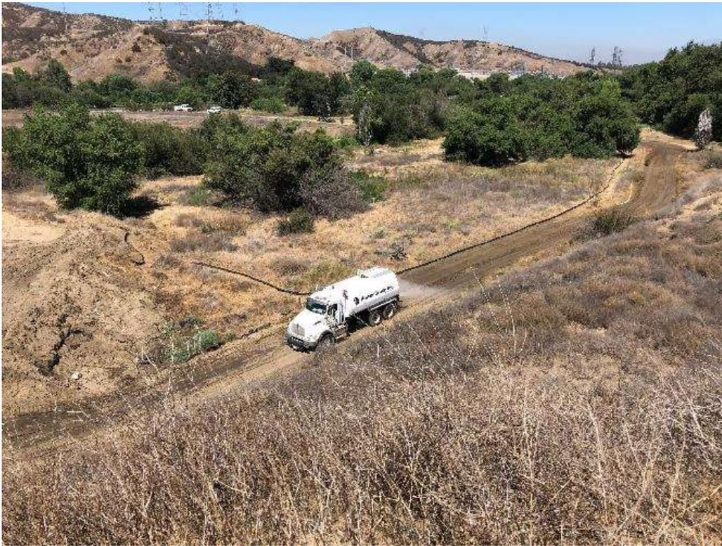
Photo 7 – Applying water to access road for Tower Site 4S60 to minimize fugitive dust (June 26, 2018).
