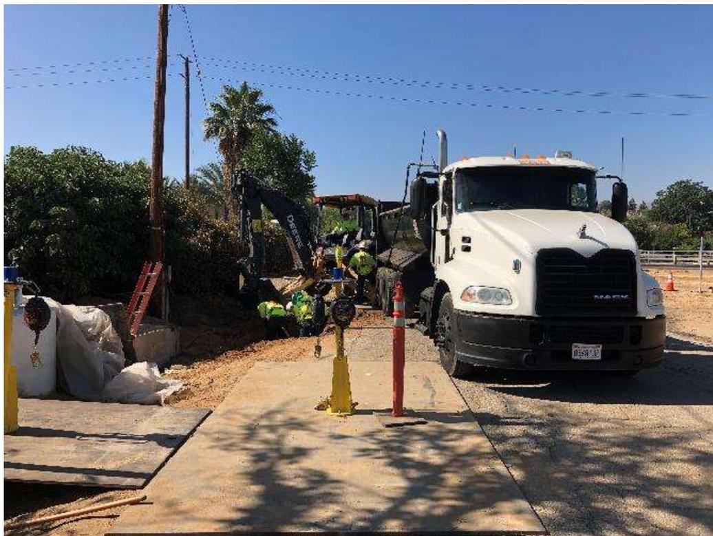
Photo 4 – Excavating for new vault at intersection of Iowa Street and Orange Avenue for the Tennessee Relocation (June 26, 2018).
