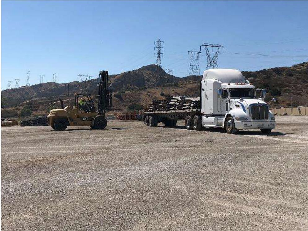
Photo 1 – Delivering stub angle steel to the Poultry MY (June 26, 2018).
