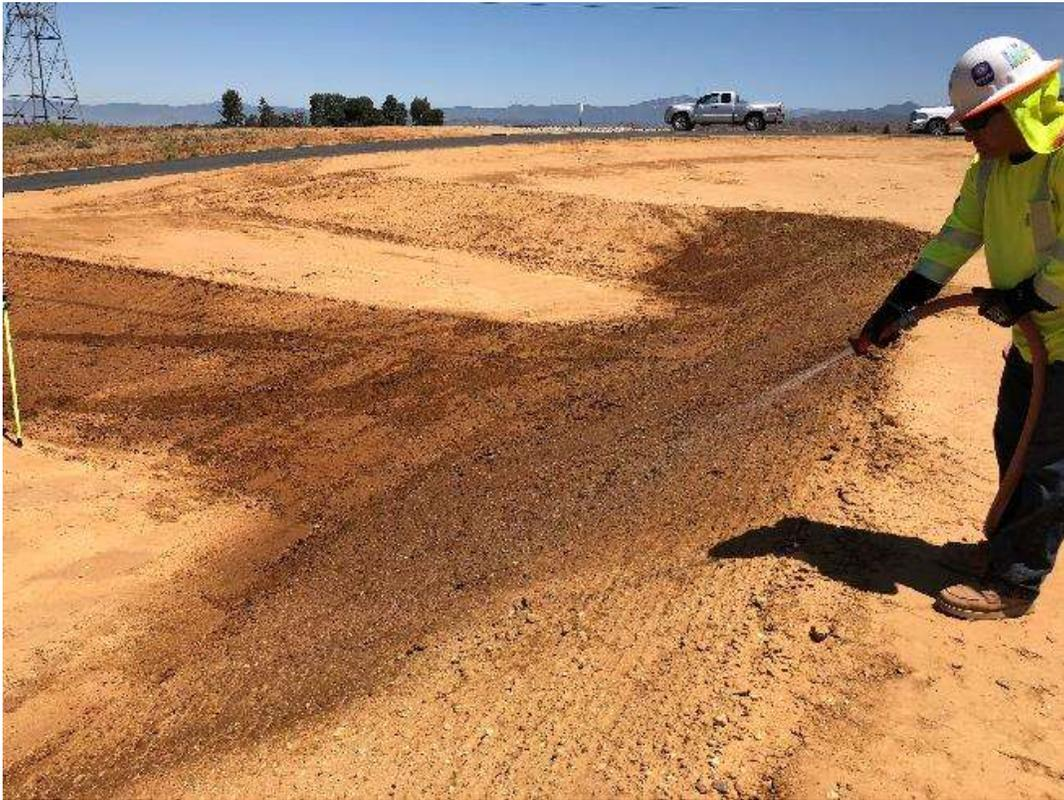
Photo 5 – Applying BMP (soil stabilizer) to slopes at Tower Site 4X47 (June 25, 2018).
