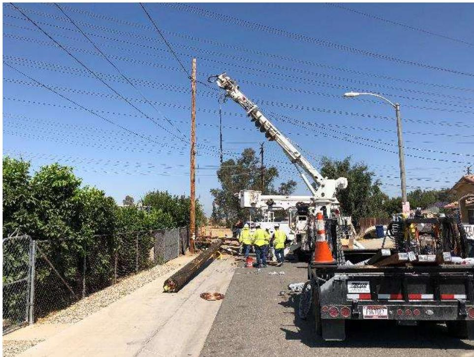
Photo 2 – Installing a new wooden pole along Juanita Street for Juanita Reconductor (June 29, 2018).
