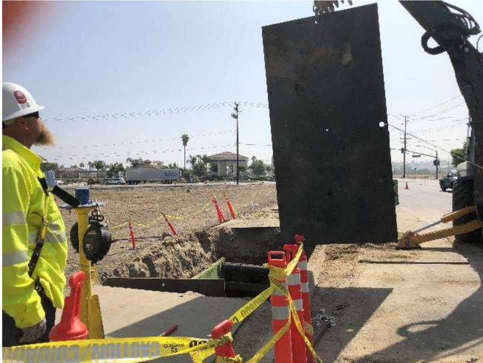
Photo 1 – Excavating underground vault along the Dental/Intern Circuit alignment (August 27, 2018).
