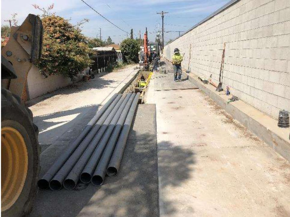
Photo 2 – Trenching and installing underground conduit along the Timoteo Relocation (August 28, 2018).
