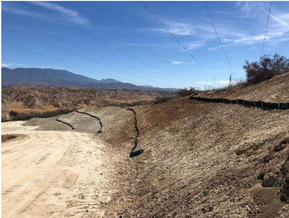
Photo 6 – Mid-slope BMPs properly installed at Site 3X19 along Segment 3 (August 30, 2018).
