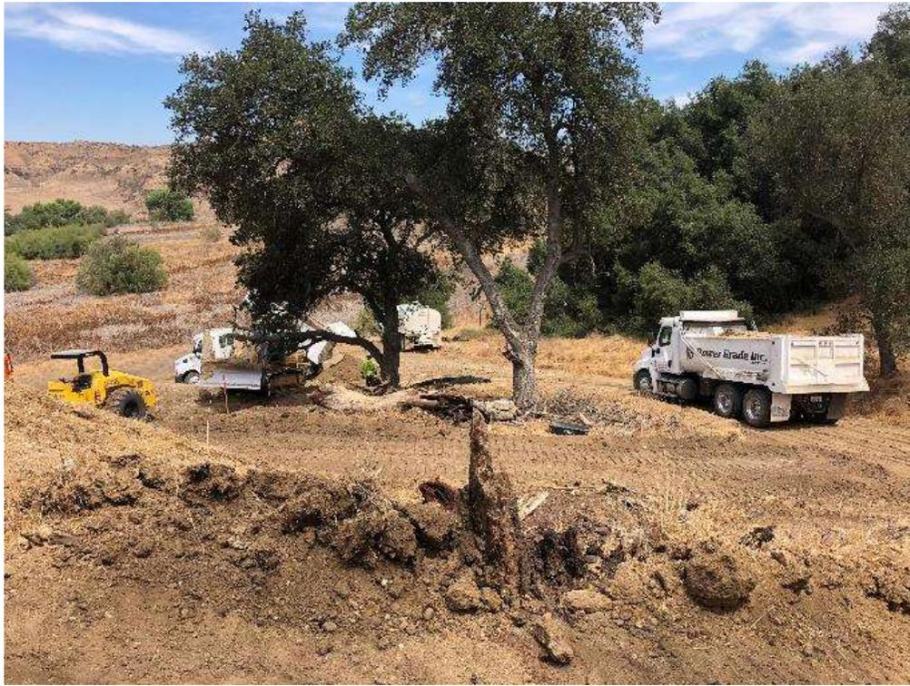
Photo 5 – Importing soils as part of grading activities at Site 4N59 along Segment 4 (August 28, 2018).
