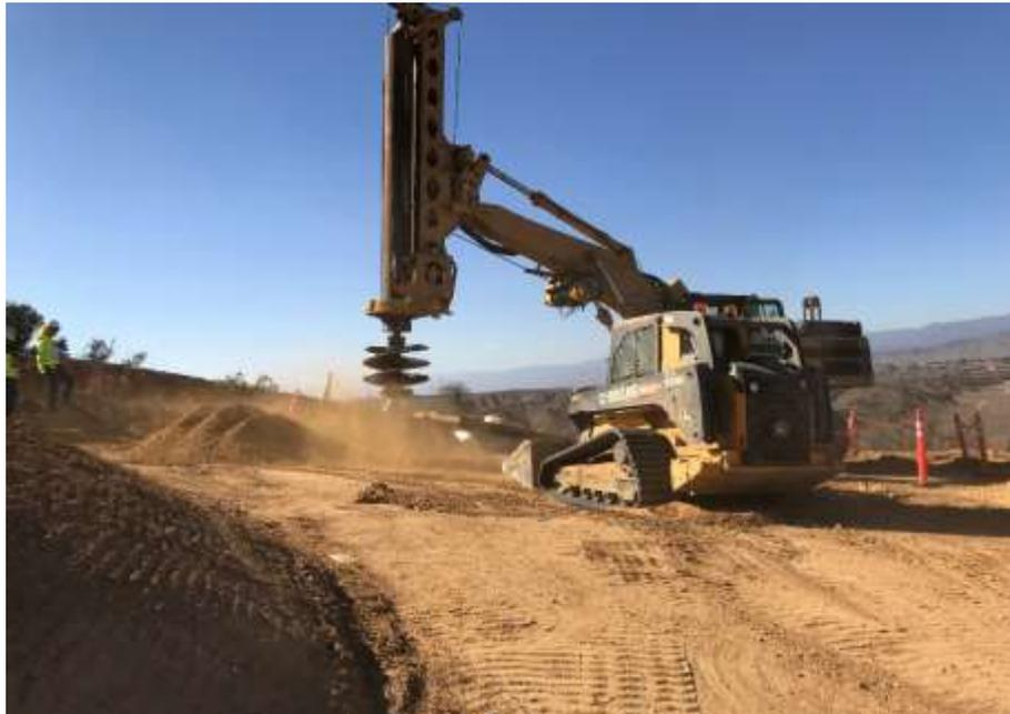
Photo 5 – Foundation drilling at Shoofly location 414. No water for fire suppression or dust abatement was on site (September 18, 2018).
