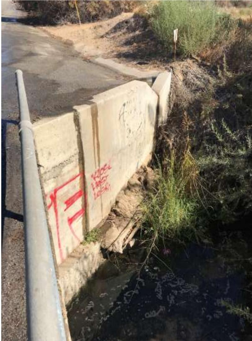
Photo 1 – Non-stormwater discharge into JD along Iowa Street from overwatering the road by subtransmission crews. No BMPs were present at the time. (September 18, 2018).
