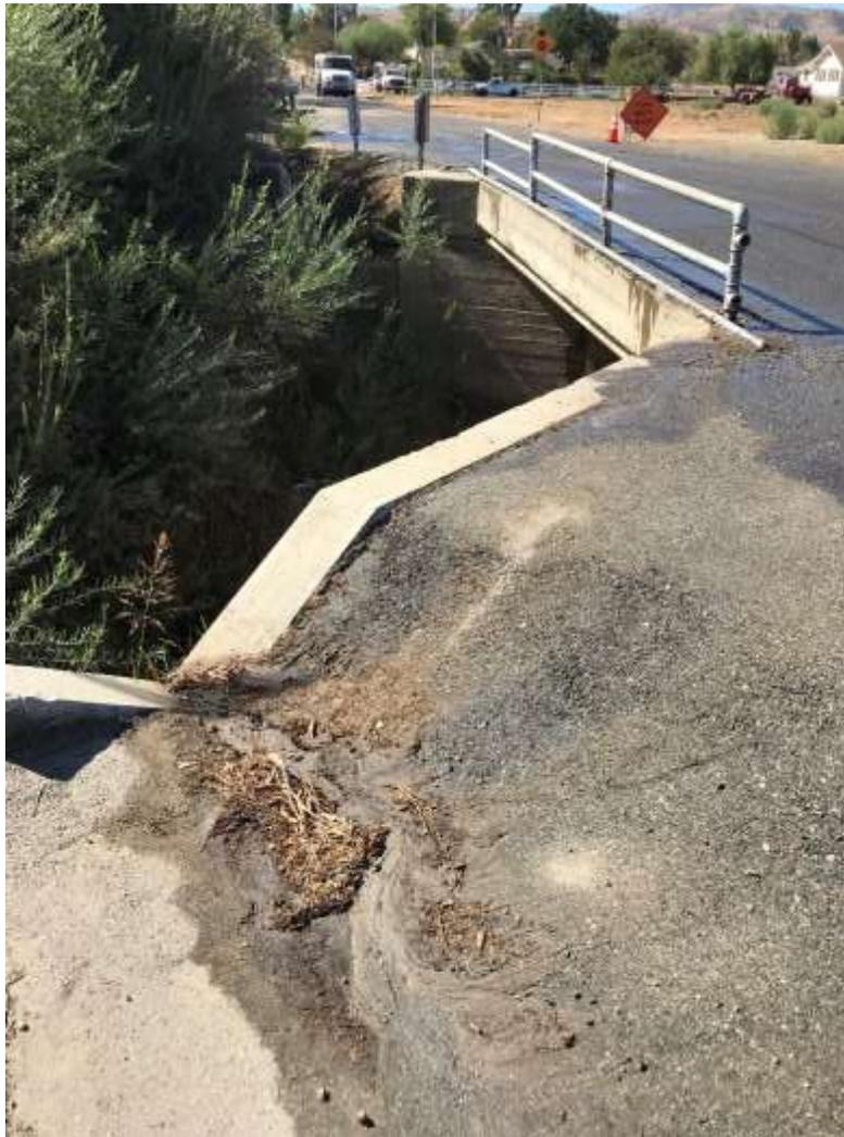
Photo 2 – Non-stormwater discharge into JD along Iowa Street from overwatering the road by subtransmission crews. No BMPs were present at the time. (September 18, 2018).
