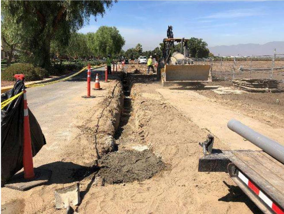
Photo 1 – Trenching and conduit installation along Mission Avenue for the Dental/Intern Circuits (September 26, 2018).
