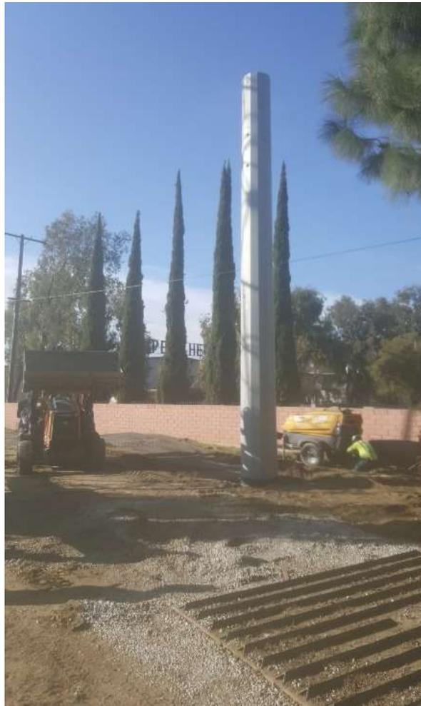
Photo 2 – Shoofly pole installation in Segment 1; part of the current outage (Move 1).
