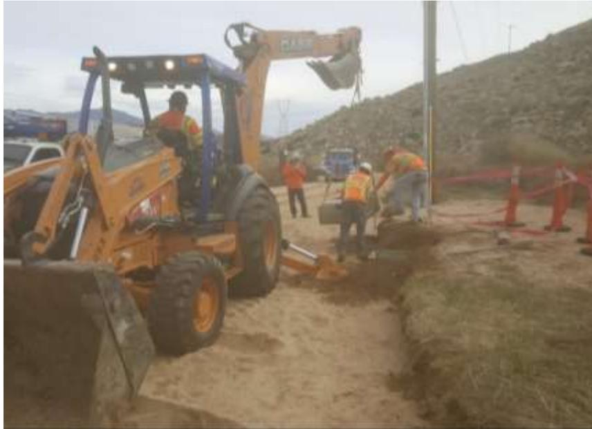
Photo 1 – Removal of the manhole exposed by erosion at Smith Creek Telecom.
