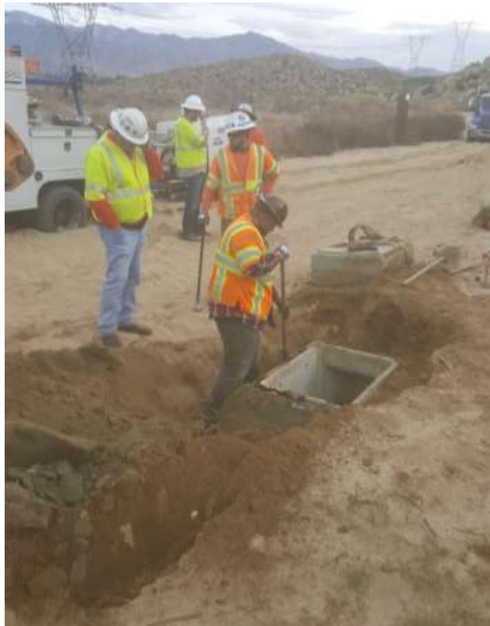
Photo 2 – Excavation of exposed manhole at Smith Creek Telecom.
