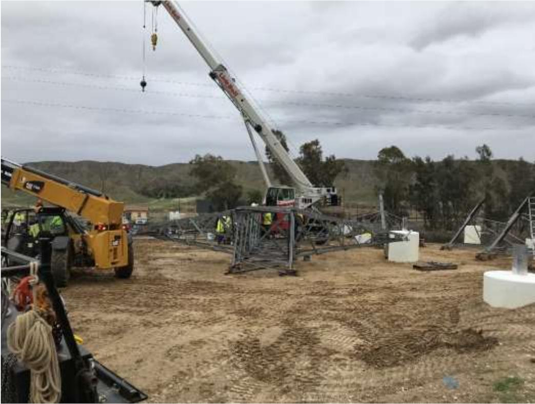
Photo 1 – Tower assembly at Site 3X22, Segment 3.
