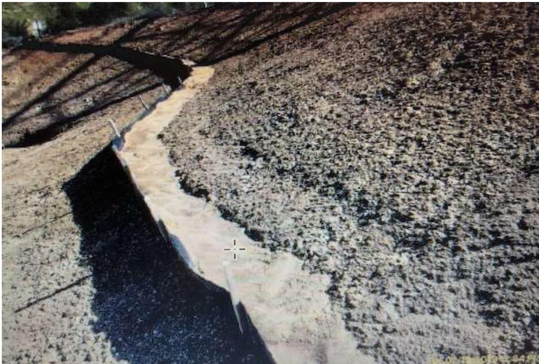
Photo 5 – Excess sediment accumulating along BMPs at Site 3X21 (Segment 3; February 19, 2019) (photo courtesy of SCE).
