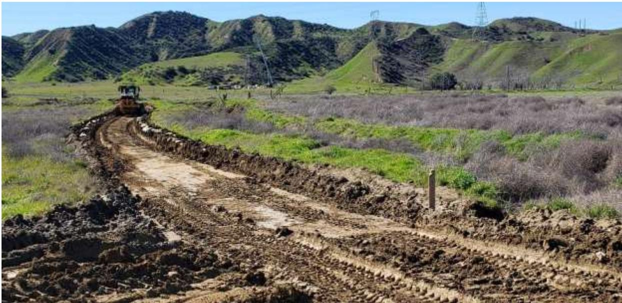
Photo 2 – Access road grading along Segment 3 (February 19, 2019).
