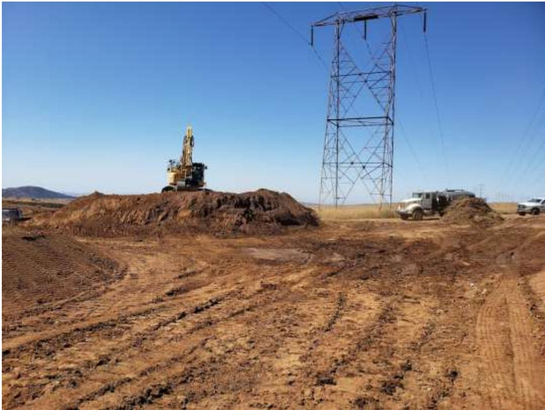
Photo 3 – Grubbing and grading activities at Construction Area 4X06, Segment 4 (September 23, 2019).
