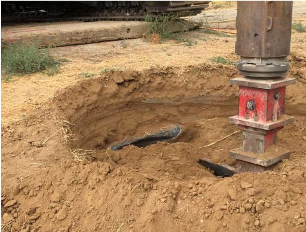
Photo 5 – Utility strike at Construction Area 2N36, Segment 2 (September 27, 2019)
