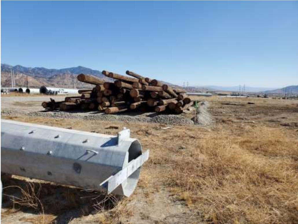
Photo 1 – Treated wood poles on cribbing with rock berm at Match MY (November 12, 2019).
