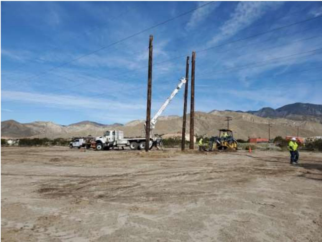
Photo 5 – Snub pole installation at Construction Area 5X01, Segment 5 (March 16, 2020).
