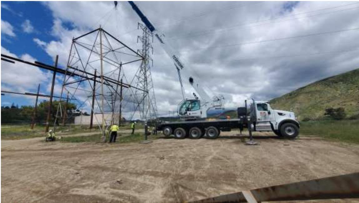
Photo 3 – Tower wreck-out at Construction Area 4X01, Segment 4 (April 11, 2020) (Photo courtesy of SCE).
