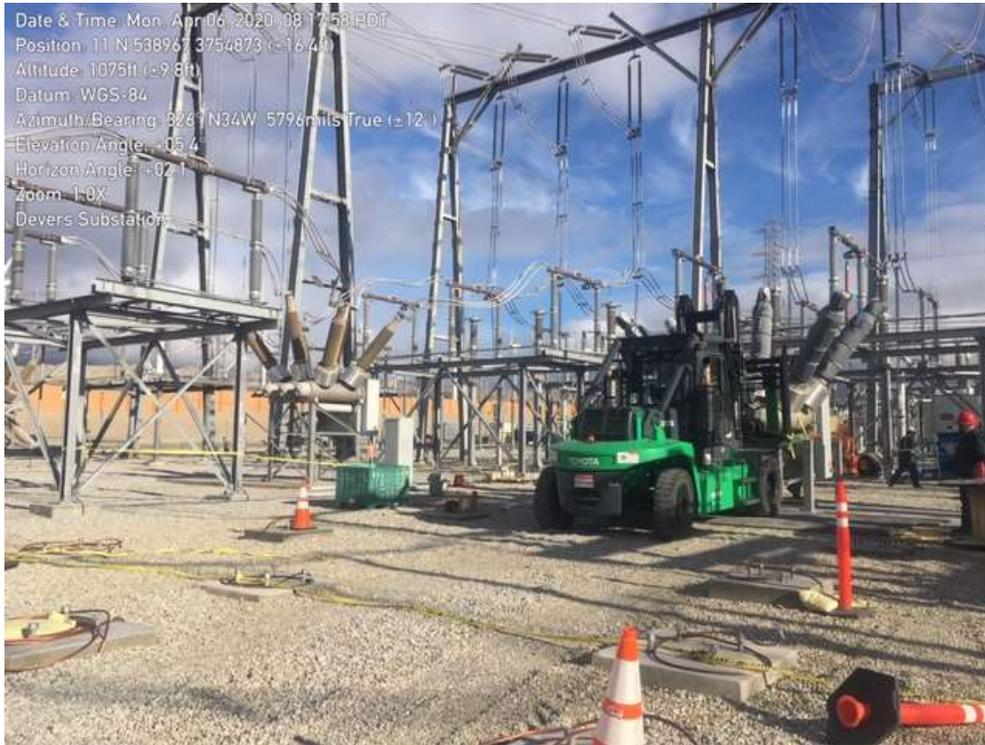
Photo 1 – Breaker installation at the Devers Substation (April 6, 2020) (Photo courtesy of SCE).
