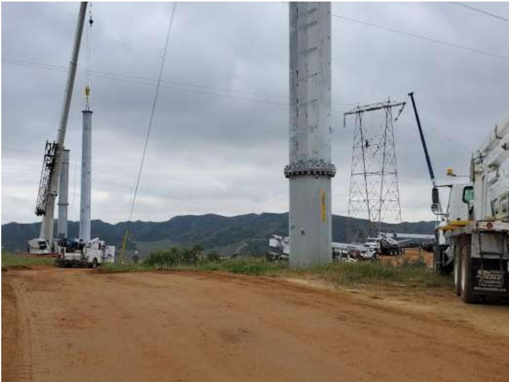
Photo 3 – Bridling conductor and installing shoofly TSP SF413 at Construction Area 4X56, Segment 4 (April 20, 2020).
