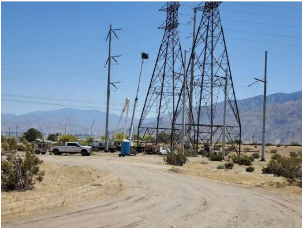
Photo 6 – Wire wreck-out activities at Construction Area 6X09-6X10, Segment 6 (May 5, 2020).
