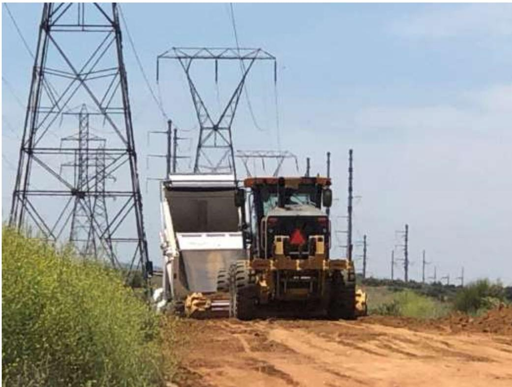
Photo 5 – Spreading spoils and access road maintenance between Construction Areas 4X51 and 4X56, Segment 4 (May 7, 2020) (Photo courtesy of SCE).
