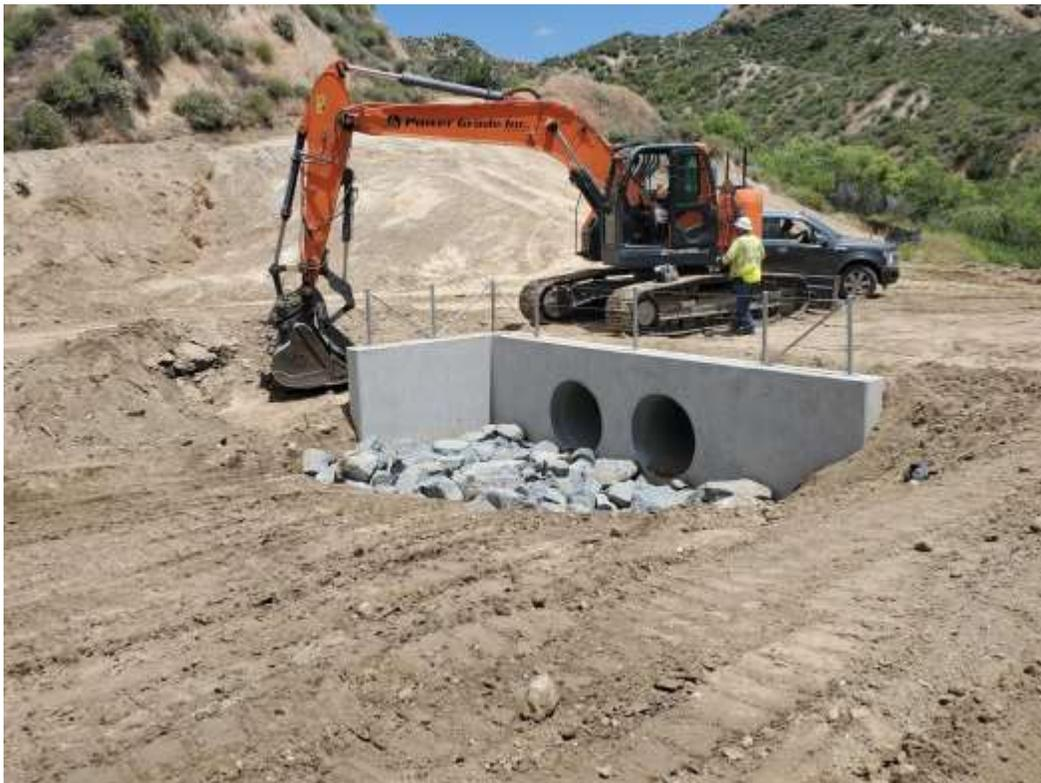
Photo 6 – Riprap installation at access road crossing to Construction Area 4X04, Segment 4 (May 19, 2020).
