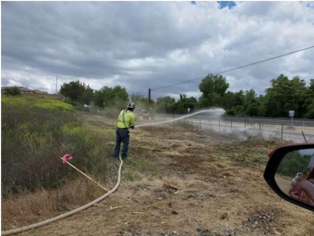
Photo 3 – Vegetation clearing at Construction Area GS-4-3S01-4S60-1-MPR-32, including watering for dust abatement, Segment 4 (May 18, 2020).
