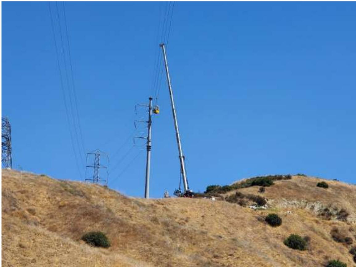
Photo 3 – Bridle conductor activities at Construction Area SF305, Segment 3 (August 10, 2020).
