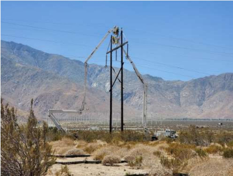
Photo 5 – Wire wreck-out activities at Construction Area 5X02 (T217), Segment 5 (August 10, 2020).
