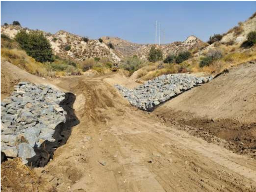
Photo 4 – Grading at wet crossing on access road to Construction Area 4X04, Segment 4 (September 16, 2020).
