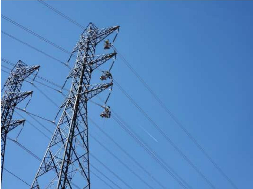
Photo 4 – Spacer installation at Construction Area 4X25, Segment 4 (October 20, 2020).
