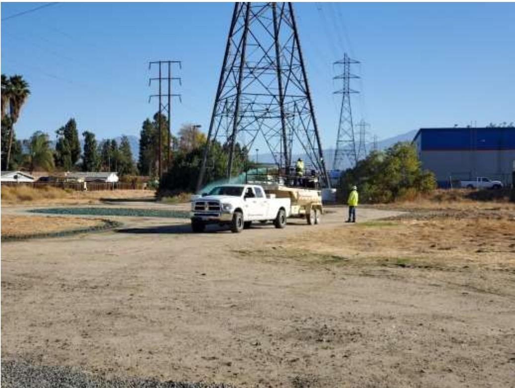
Photo 2 – Hydroseed application at Construction Area 2N35, Segment 2 (December 15, 2020).
