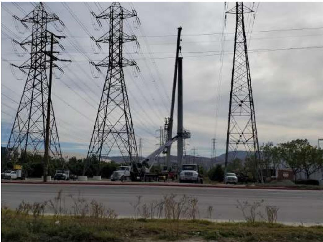
Photo 2 – Shoofly tower wreck-out at Construction Area 1X25, Segment 1 (January 13, 2021).
