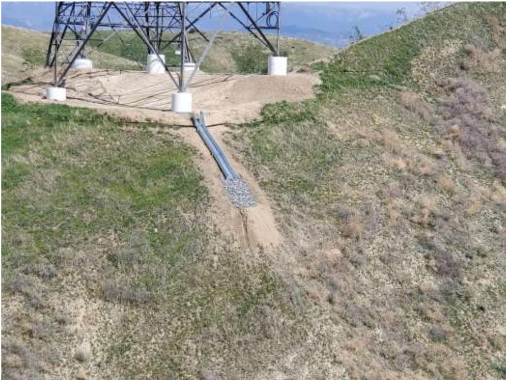
Photo 7 - Erosion downslope of MAC drain at Construction Area 3X65, Segment 3 (March 16, 2021).
