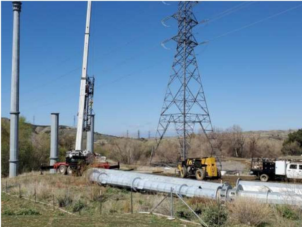
Photo 3 – Shoofly tower wreck-out at Construction Area 4S60, Segment 4 (March 16, 2021).
