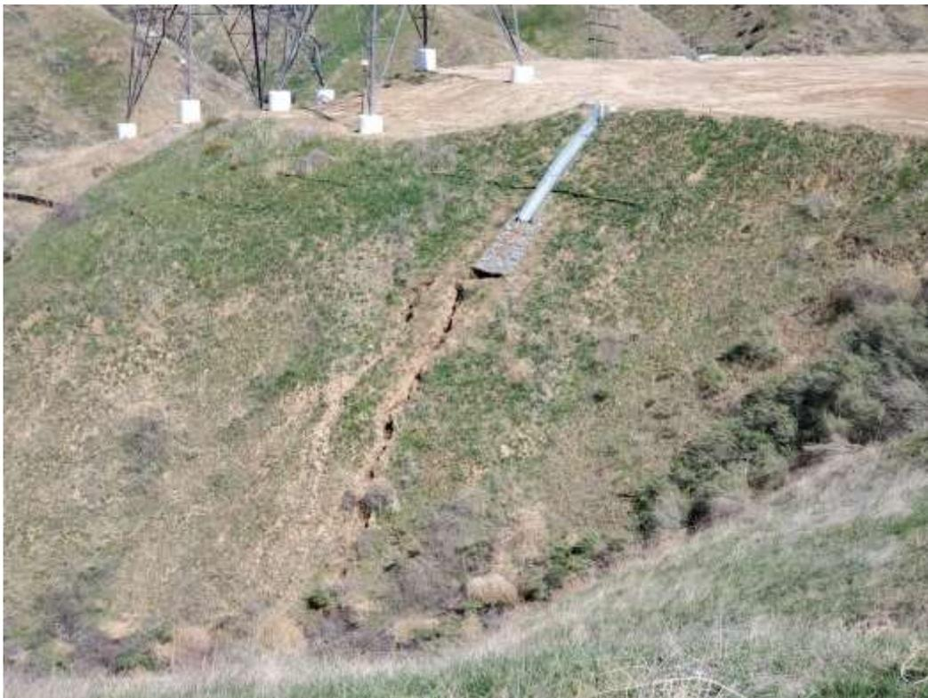
Photo 6 – Erosion downslope of MAC drain at Construction Area 3X64, Segment 3 (March 16, 2021).
