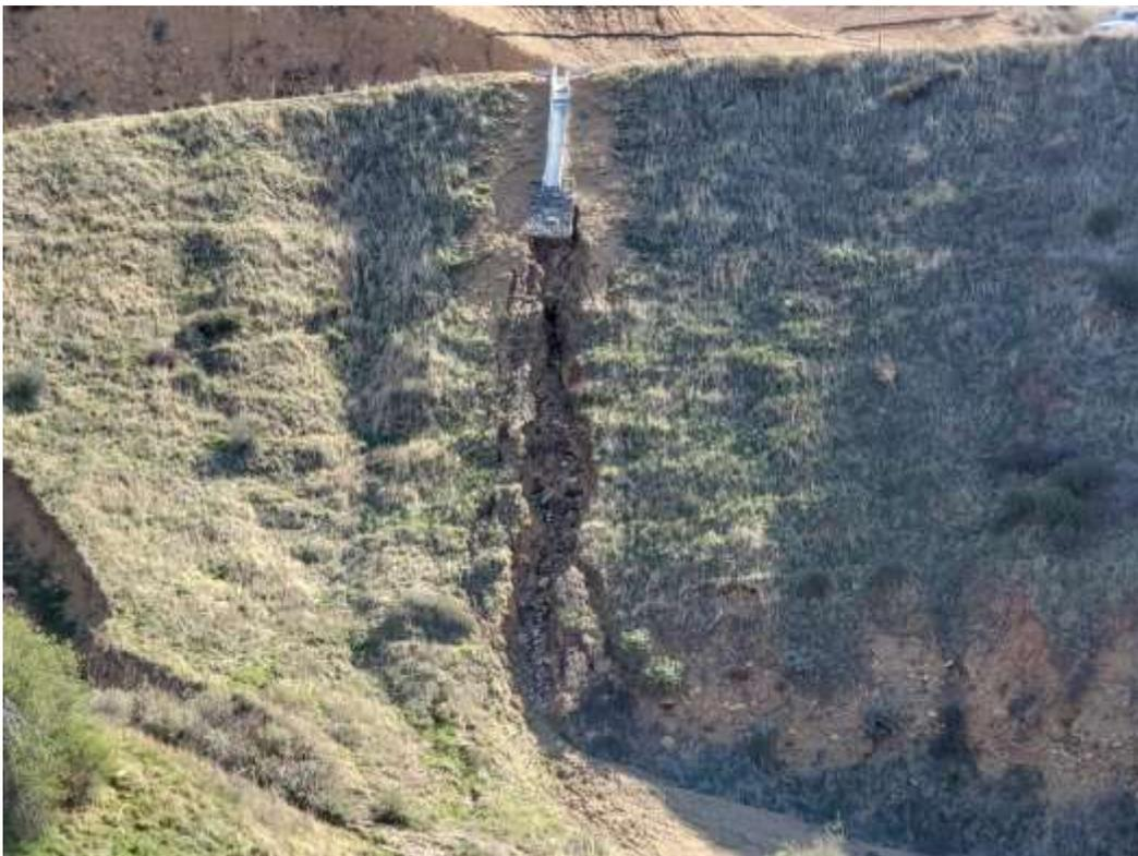
Photo 8 - Erosion downslope of MAC drain at Construction Area 4X06, Segment 4 (March 19, 2021).
