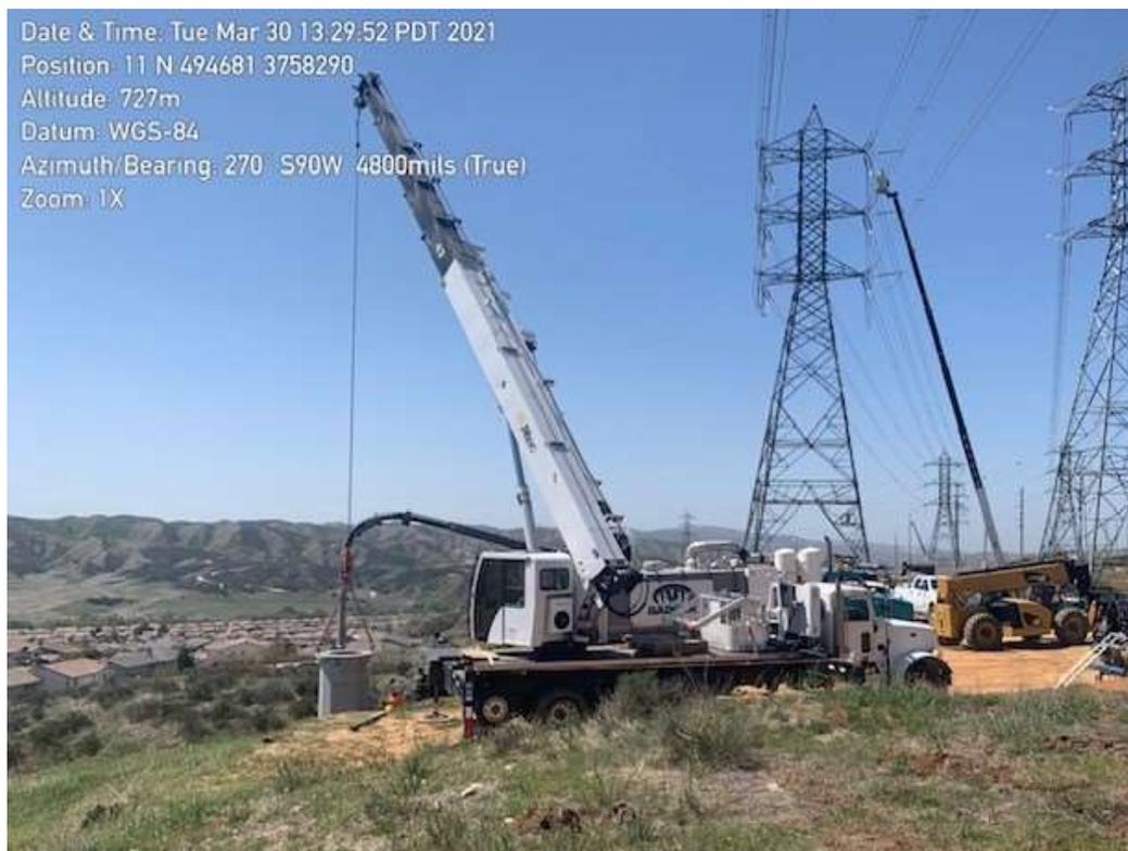
Photo 4 – Shoofly base removal at Construction Area 4X56, Segment 4 (March 30, 2021) (Photo courtesy of SCE).
