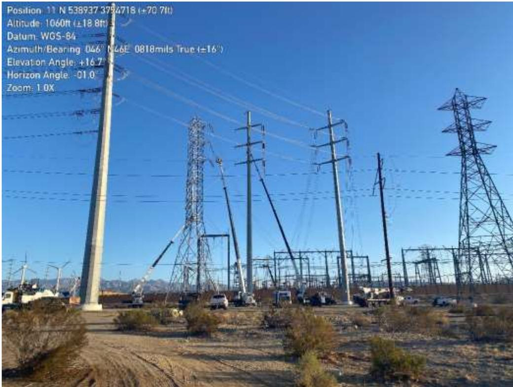
Photo 5 – Wire wreck-out activities at Construction Area 6X08, Segment 6 (April 1, 2021)
