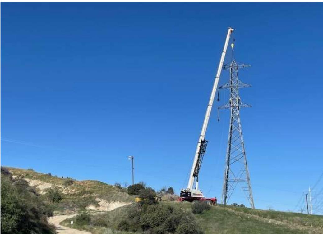
Photo 2 – Tower wreck-out activities at Construction Area 3X25, Segment 3 (March 31, 2021) (Photo courtesy of SCE).
