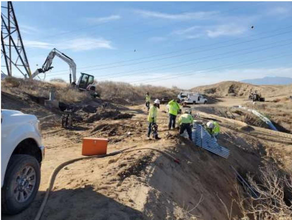
Photo 2 – MAC drain installation and foundation removal at Construction Area 2N12, Segment 2 (November 15, 2021).
