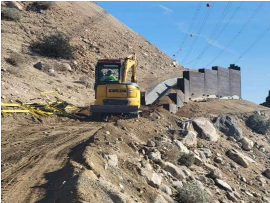
Photo 6 – V-ditch dissipator installation at Construction Area 6N30, Segment 6 (January 4, 2022) (Photo courtesy of SCE).
