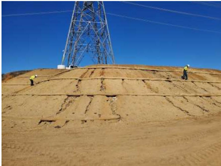
Photo 4 – Erosion repair at Construction Area 4X06, Segment 4 (February 3, 2022).
