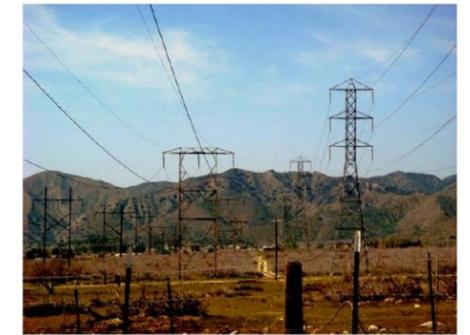
(average height 83 feet for single-circuit towers and 140 feet for double circuit towers) and installation of 108 towers (average height 144 feet).
