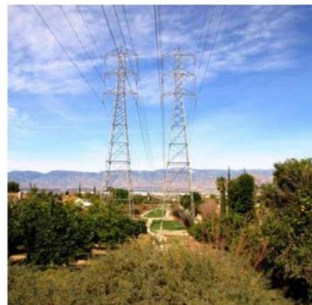
Transmission line work within Segment 1 would include removal of approximately 45 double circuit towers (average height 136 feet) and installation of 61 towers (average height 135 feet), within the existing ROW.
