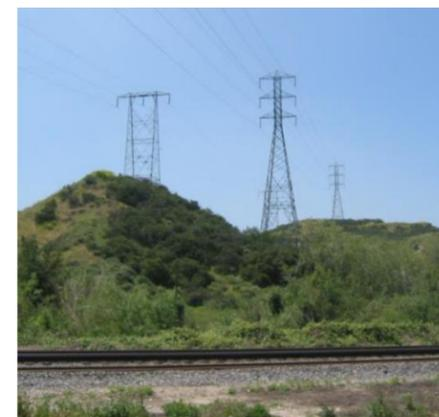
Segment 3 includes three separate sets of existing towers that would be removed and replaced with two sets of new 220 kV double circuit towers. Project work within Segment 3 would include removal of 116 towers (average height 86 feet for single-circuit towers and 139 feet for double-circuit towers) and installation of 133 towers (average height 143 feet).
