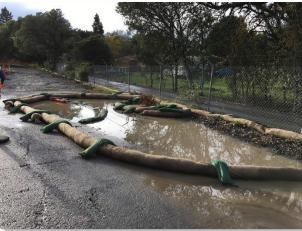
Figure 6. Drainage inlets on north side of site, view west, December 9, 2016
