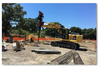
Figure 15. Augering holes for perimeter wall piers at Substation, view northwest, June 13, 2017
