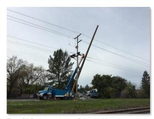
Figure 24. Replacing pole along Fulton No. 1 line, view west, January 29, 2018
