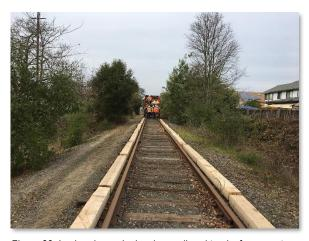
Figure 23. Laying down planks along railroad tracks for crane to drive over, view north, December 19, 2017
