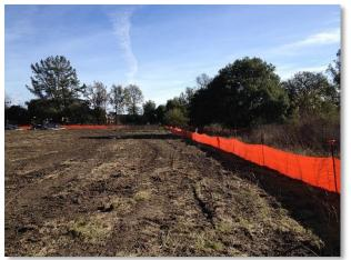
Figure 5. Silt fence-ESA fence installed on west and south sides, view south, November 28, 2016
