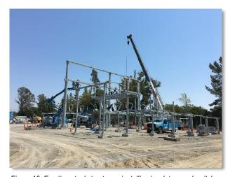
Figure 16. Erecting steel structures, installing insulators and switches, view southeast, August 1, 2017
