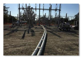
Figure 19. HDD conduit ready to be pulled back through hole, view west, October 31, 2017
