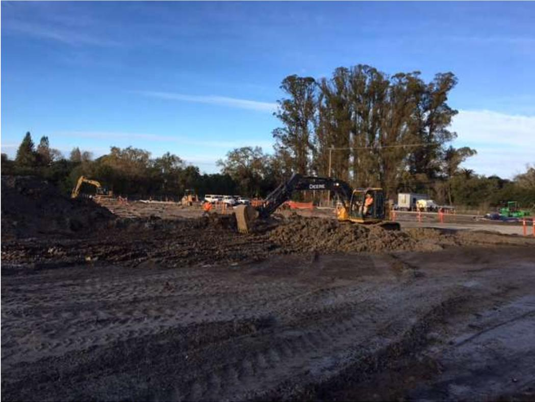
Figure 1 – Excavating soil in central area of substation site, December 12, 2016.
