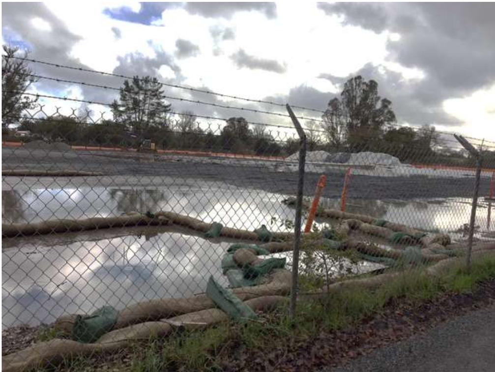
Figure 2 – Drainage inlets protected with BMPs on north side of substation site – view southwest, January 20, 2017.
