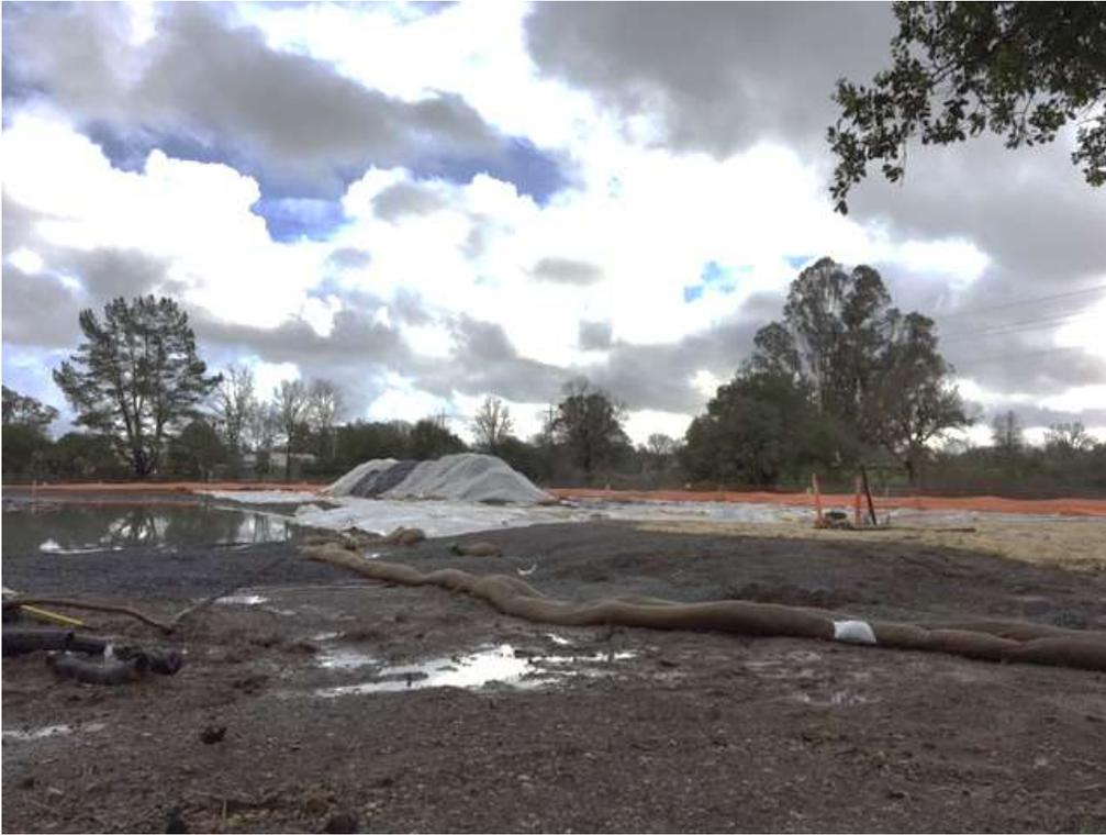
Figure 1 – Spoil piles covered with plastic and bare areas covered with straw at substation site – view southwest, January 20, 2017.
