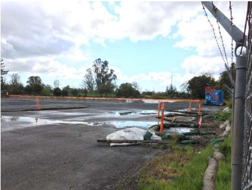
Figure 2 – Drainage inlets protected with BMPs on north side of substation site – view west, March 22, 2017.
