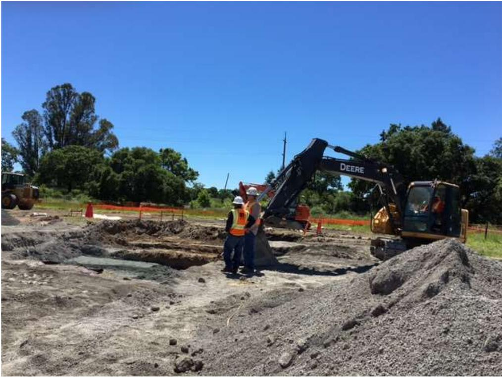
Figure 3 – Switchgear excavation at substation site – view west, May 2, 2017.
