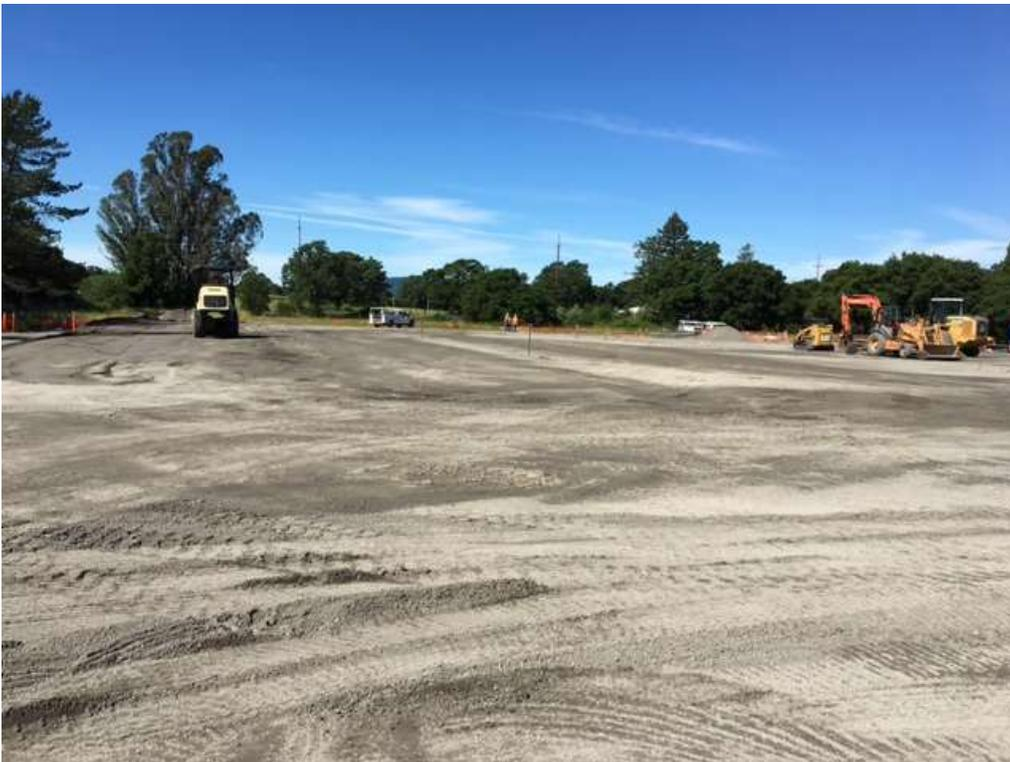
Figure 2 – Spreading and compacting base rock at substation site – view west, May 4, 2017.
