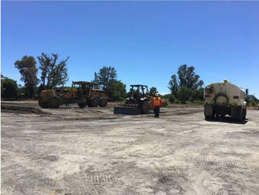
Figure 1 – Spreading and compacting base rock at substation site – view southwest, May 2, 2017.
