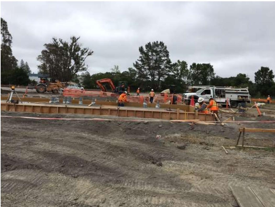
Figure 2 – Switchgear foundation work at the substation site – view south, May 10, 2017.
