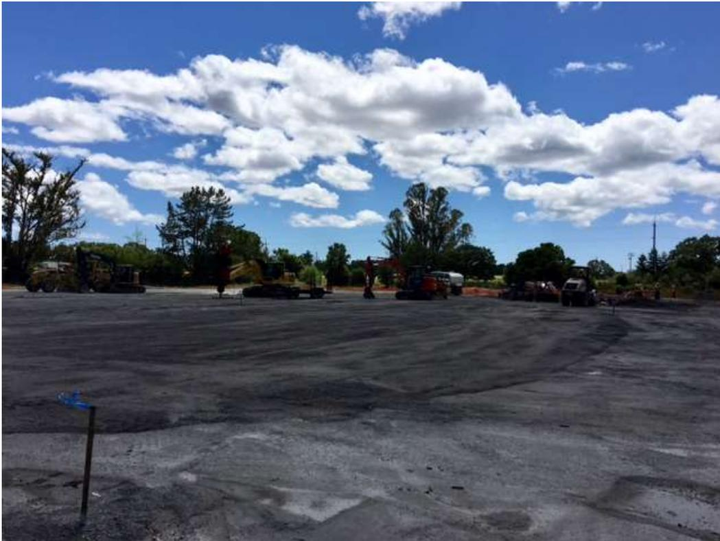
Figure 3 – Spreading and compacting additional base rock for pad at substation site – view west, May 12, 2017.
