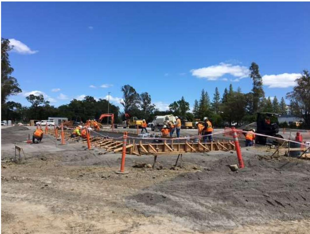
Figure 4 – Switchgear foundation work at substation site – view east, May 12, 2017.
