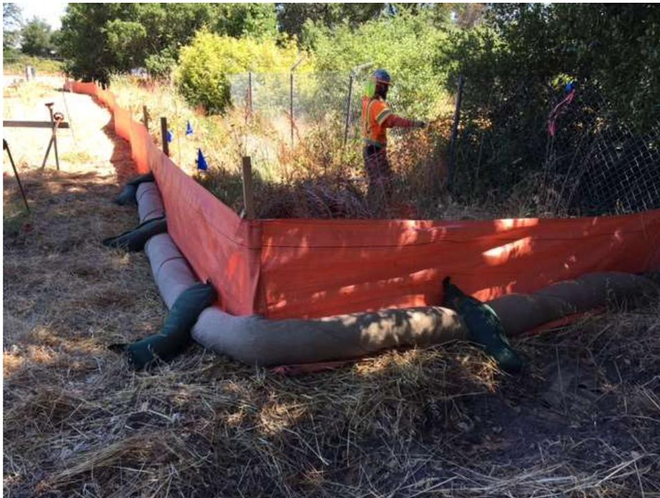
Figure 2 – Relocation of silt fence in northwest corner of substation site – view south, June 26, 2017.
