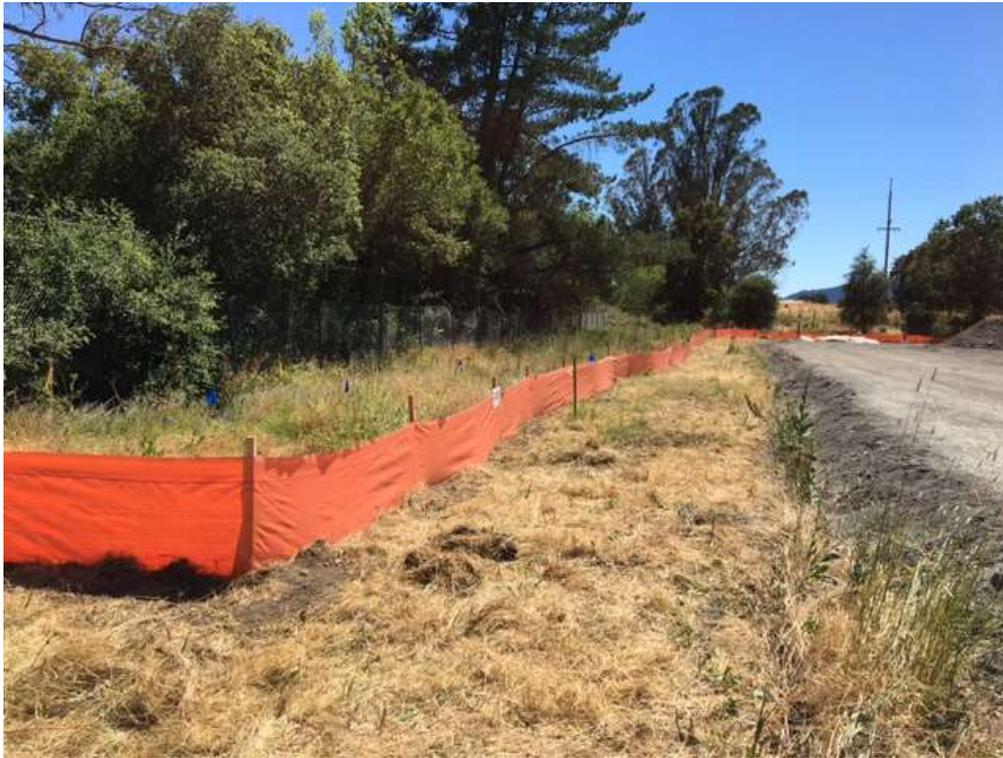
Figure 3 – Relocation of silt fence on south side of substation site – view west, June 26, 2017.
