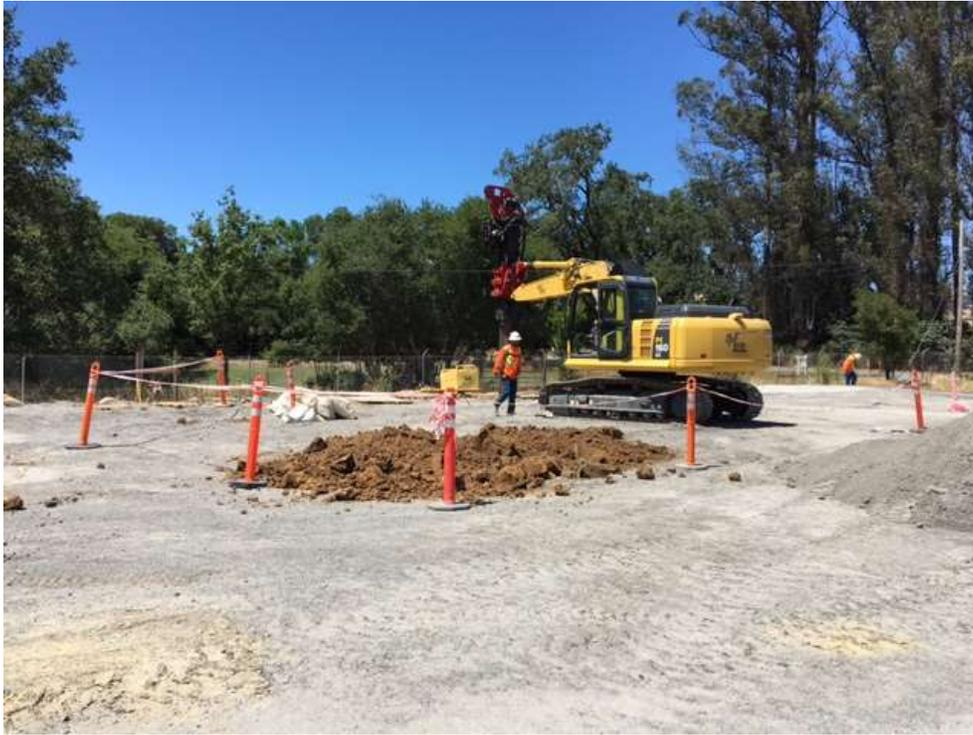
Figure 1 – Drilling foundation holes for perimeter wall piers on north side of substation – view northeast, June 26, 2017.
