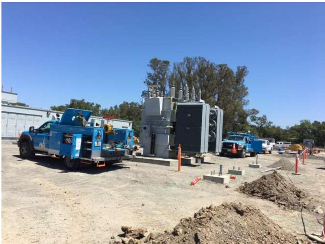
Figure 2 – Welding transformer to foundation pad – view east-northeast, July 12, 2017.
