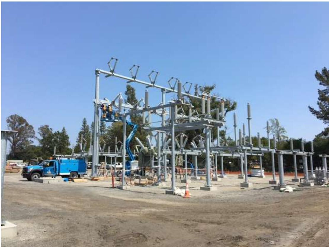
Figure 4 – Installation of switches on dead-end structures – view southeast, August 10, 2017.
