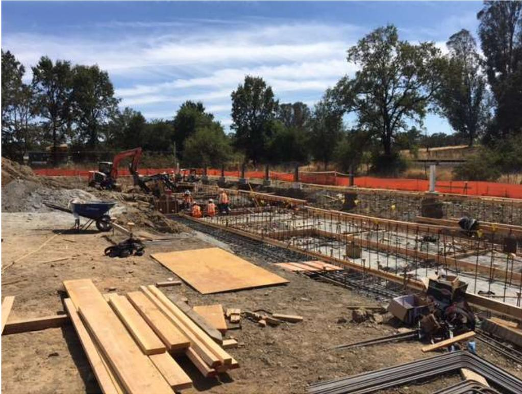
Figure 1 – Tying rebar in the SPCC ponds on west side of site – view southwest, August 24, 2017.
