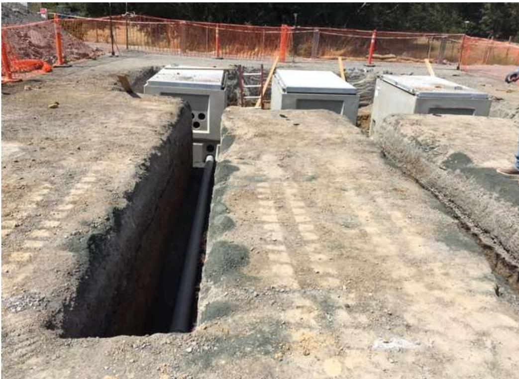
Figure 2 – Installing conduit to pull boxes set on northern perimeter – view north, August 24, 2017.
