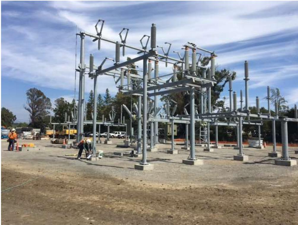
Figure 3 – Installation of switches and insulators on dead-end structures – view southeast, August 24, 2017.
