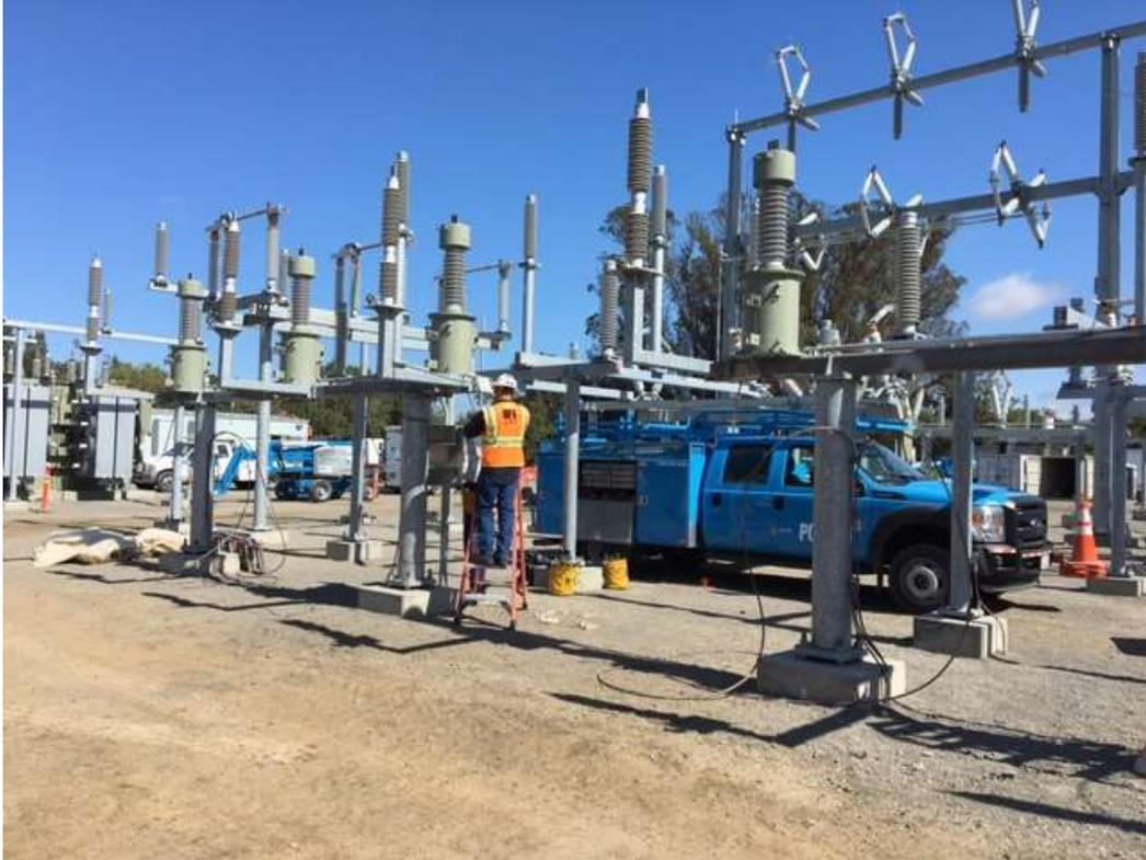
Figure 3 – Installing switches and insulators on dead-end structures – view northeast, September 14, 2017.
