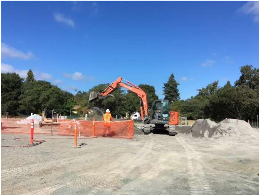
Figure 1 – Backfilling conduit trenches – view north, September 14, 2017.
