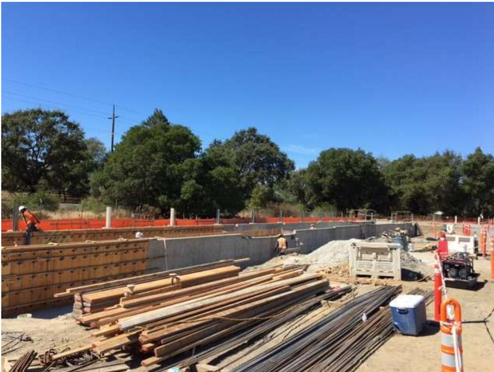
Figure 2 – Installing rebar and wall forms for the SPCC pond – view northwest, September 27, 2017.
